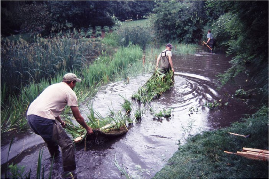
Aquatic plants being installed at Willow Pond's emergent shelf, 2005.
